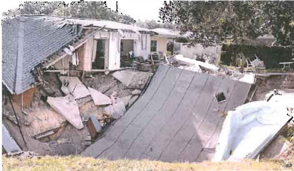
Figure 5.11 – Sinkhole Collapse of a House
